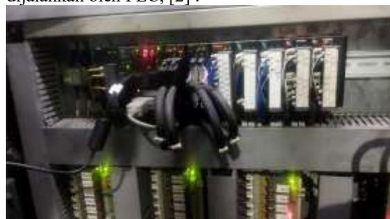
Gambar 4. PLC Omron CJ2M CPU33
